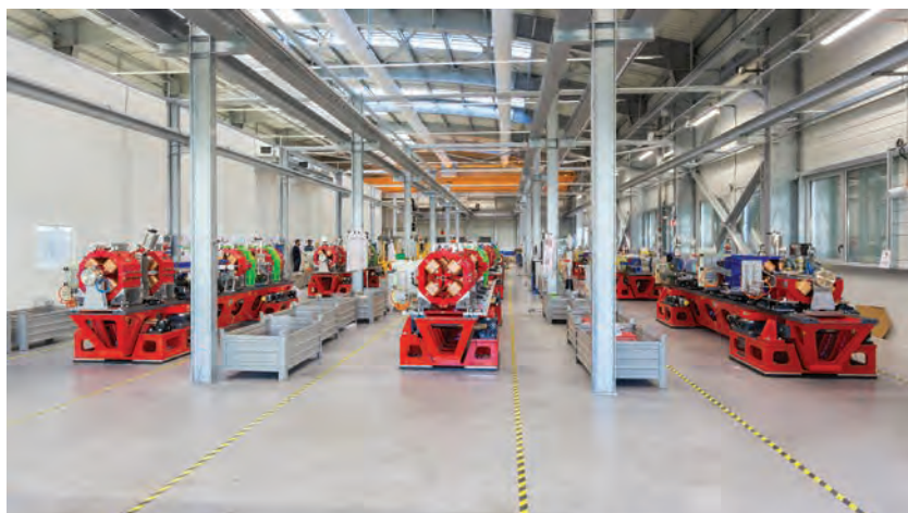
Fig. 1: The production line of girders in assembly building ESRF 01. By the end of 2018, most of the EBS girders were assembled, ready for installation in the storage ring in spring 2019.
